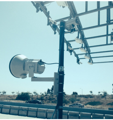
Figure 2: Front Camera and Illuminator (I-15 and Miramar Way)
